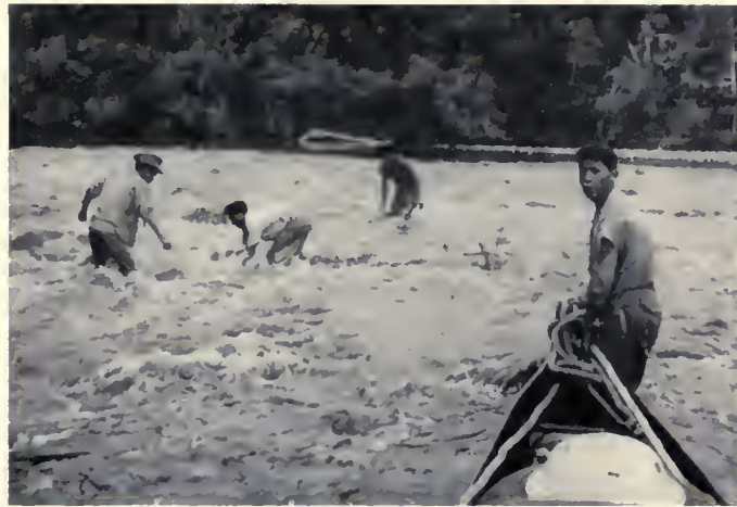
CLEARING A CHANNEL
