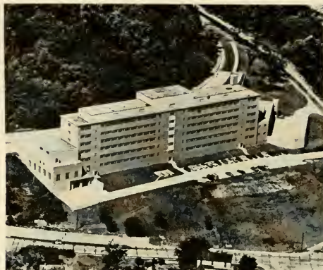
ROBERT A. TAFT SANITARY ENGINEERING CENTER
