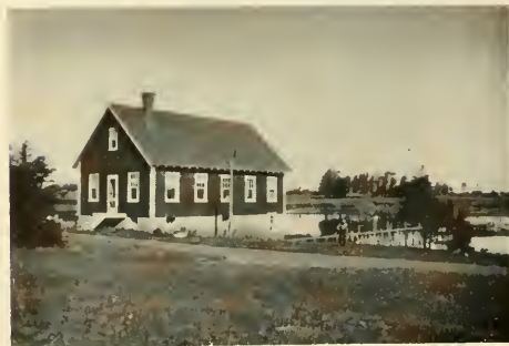
BIOLOGICAL SUB-STATION, ELLERSLIE
