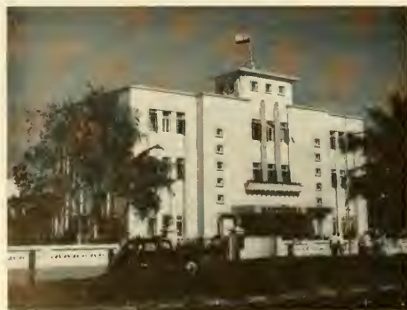
TARAPOREVALA AQUARIUM AND MARINE BIOLOGICAL RESEARCH STATION, BOMBAY
