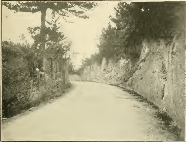
Figure 12.—Road Cutting near Hamilton.
