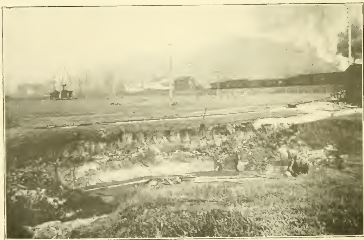
FIG. 2. Near view of cave-in at "Well No. 69," Mathieson Alkali Works, Saltville, Virginia.
