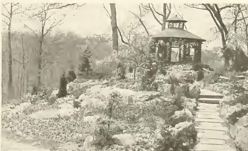
Rockgarden at "Lindenhurst." May effect a year after construction.
