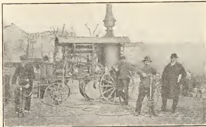
PNEUMATIC TAMPER FOR PAVING BLOCKS.
