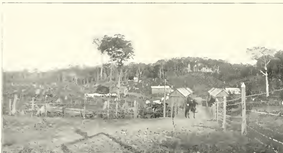
"DEL CORTE," LABORERS' CAMP AND CLEARING.
