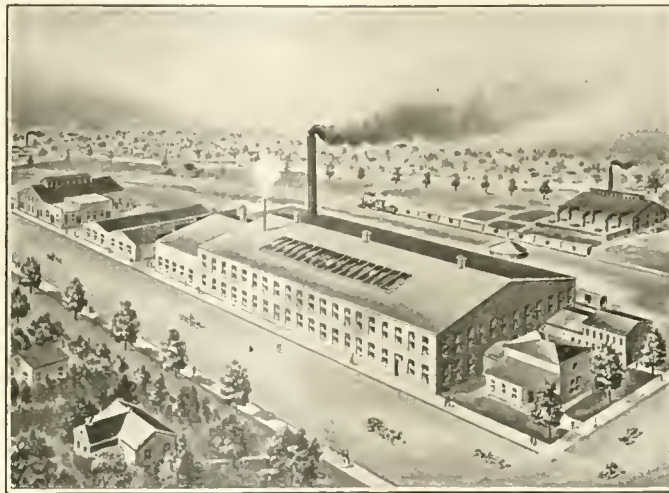
FIRESTONE TIRE AND RUBBER CO.'S FACTORY.
