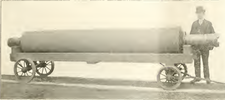
RUBBER COVERED ROLLER FOR PAPER MAKING MACHINE.
