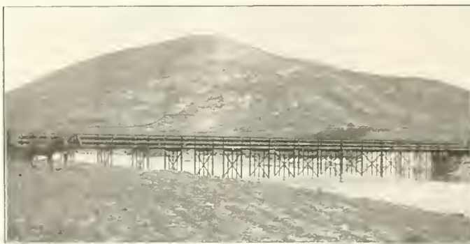
BRIDGE BUILT WITH RAILROAD RAILS.
