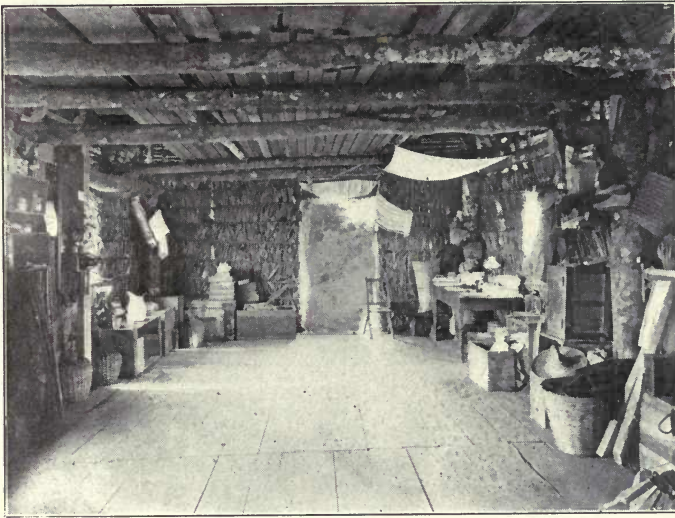
RUBIO.—INTERIOR OF TEMPORARY OFFICE.
