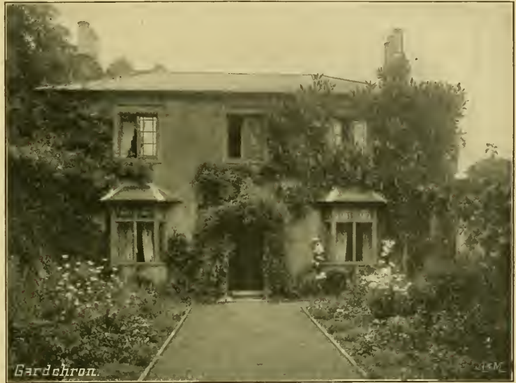
FIG. 15.—NUNEHAM PARK: THE GARDENER'S COTTAGE.
