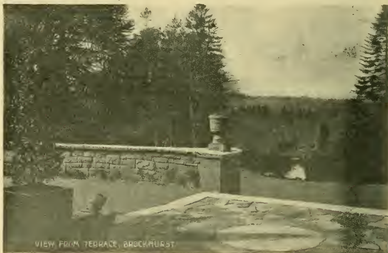
FIG. 118.—BROCKHURST, EAST GRINSTEAD.
