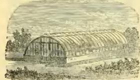
**LASCELLES' PATENT BENT WOOD CONSERVATORIES and GREENHOUSES**—All Gardeners know that Wood is better than Iron for Plant Growing, and by the above system a handsome curved lighter can be erected as cheaply as a plain straight one. The curved house is more durable, stronger, higher in construction, and no bent glass is required. **W. H. LASCELLES**, 172, Bonhill Row, London, E.C., will supply Drawings and Estimates free of charge.
