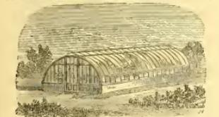
**LASCELLES' PATENT BENT WOOD CONSERVATORIES and GREENHOUSES.**—All Gardeners know that Wood is better than Iron for Glass Growing, and by the above system a handsome curved house can be erected as cheaply as a plain straight one.
