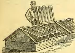
This is the Practical Gardener's and Nurseryman's favourite frame, now largely used for storing the great quantities of bedding plants in winter, and is much used for growing Melons, &c. This is suitable for building on brickwork, as shown by section of No. 64.
