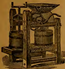
Cider Mills—with wooden crushing rollers.
