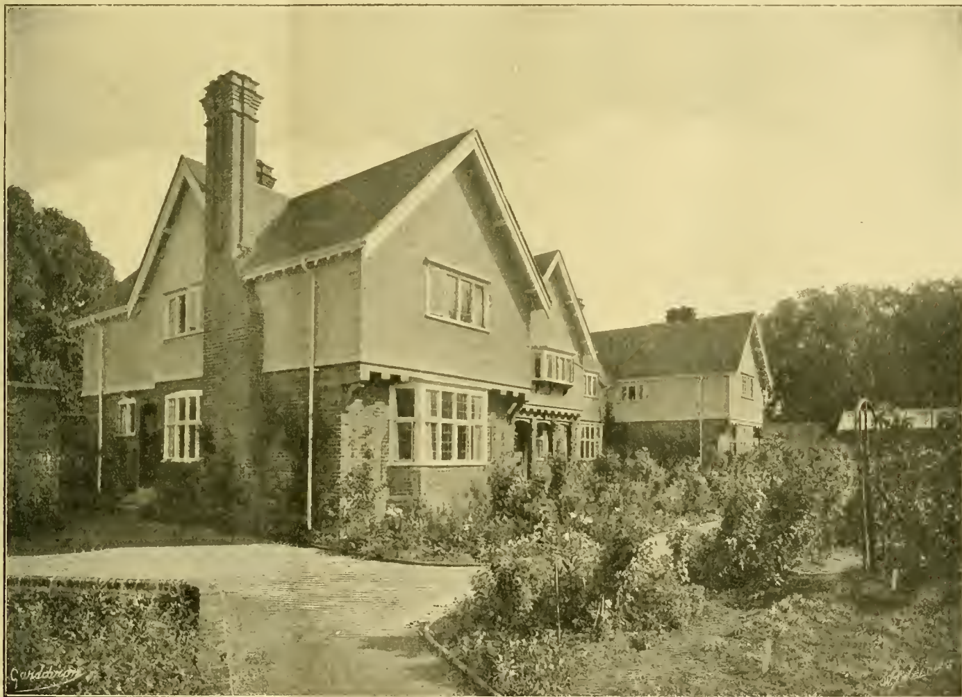
FIG. 142.—THE NEW BOTHY AT TRING PARK GARDENS.
