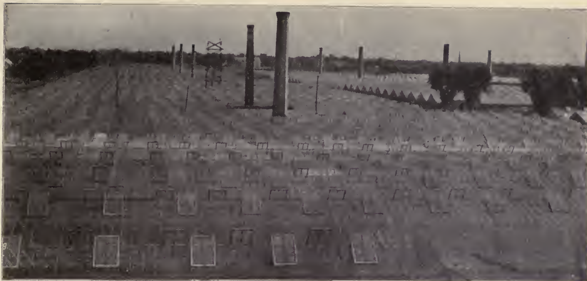
Ventilation Sashes Alternating on the Two Sides of the Ridge.
