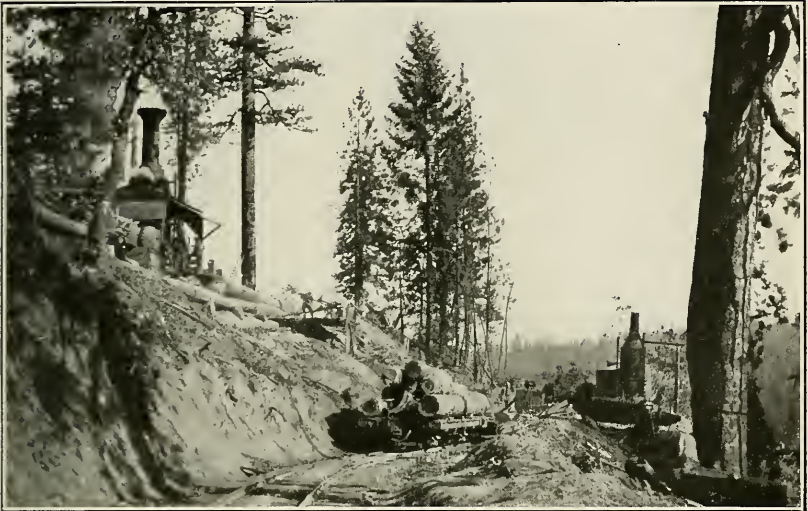
FIG. 1.—A 12 BY 14 YARDER AT A RAILROAD LANDING IN THE SUGAR PINE REGION. Logs yarded in long lengths and bucked in chute. Separate loading engine below track.
