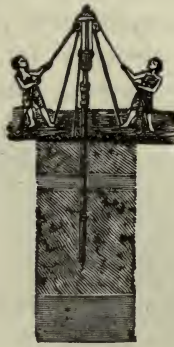
FIG. 46.--MANNER OF FIXING NUBIAN TUBE-WELLS.
