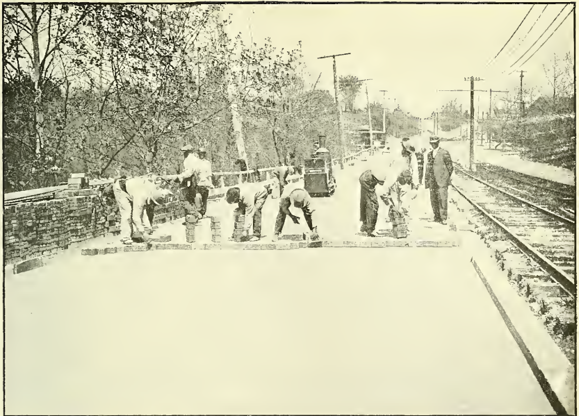
FIG. 1.—LAYING THE BRICK.
