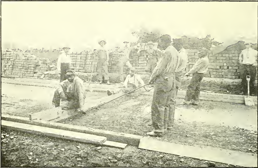
FIG. 1.—FINE GRADING.
