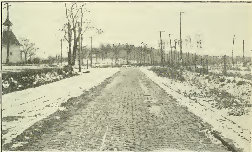
FIG. 2.—FAILURE OF BRICK ROAD NEAR MANSFIELD, OHIO, DUE TO DEFECTIVE CONSTRUCTION AND HEAVY MOTOR-TRUCK TRAFFIC.
