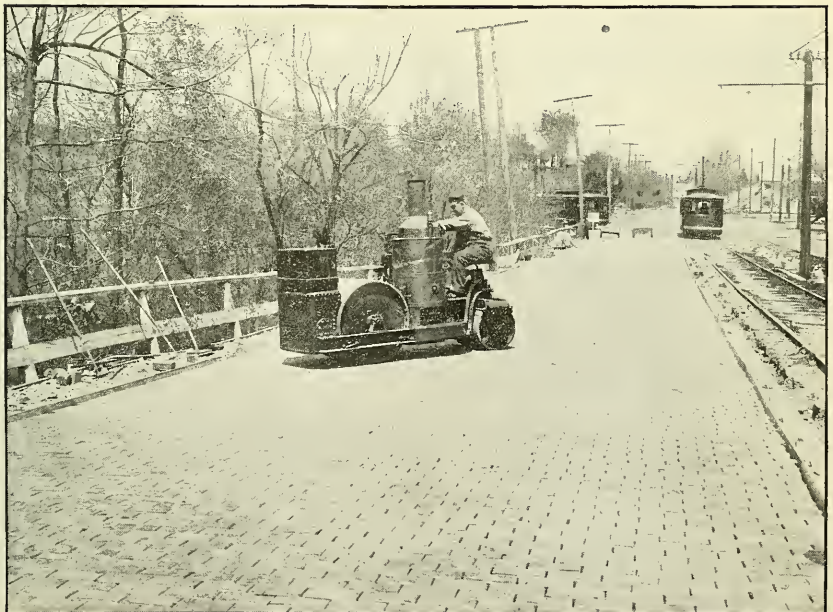
FIG. 2.—ROLLING THE PAVEMENT.
