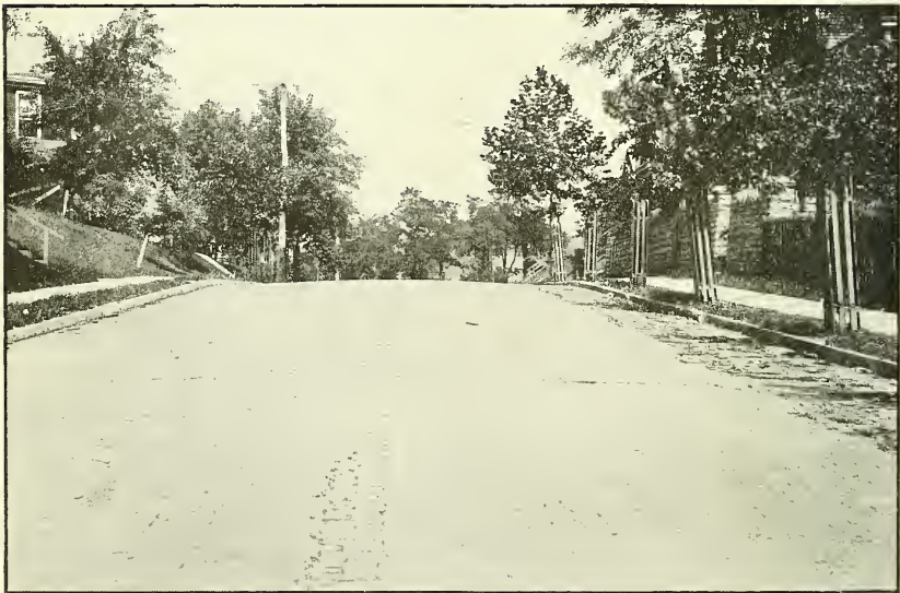
FIG. 2.—GROUT-FILLED BRICK PAVEMENT, HAVING LONGITUDINAL JOINTS IN CENTER AND OCCASIONAL TRANSVERSE JOINTS FILLED WITH SOFT FILLER. Unightly appearance at right caused by widening roadway.
