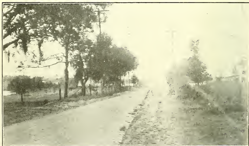
FIG. 2.—BRICK ROAD AT ORLANDO, FLA., SHOWING DISPLACEMENT OF MARGINAL BRICK DUE TO ABSENCE OF CURB.
