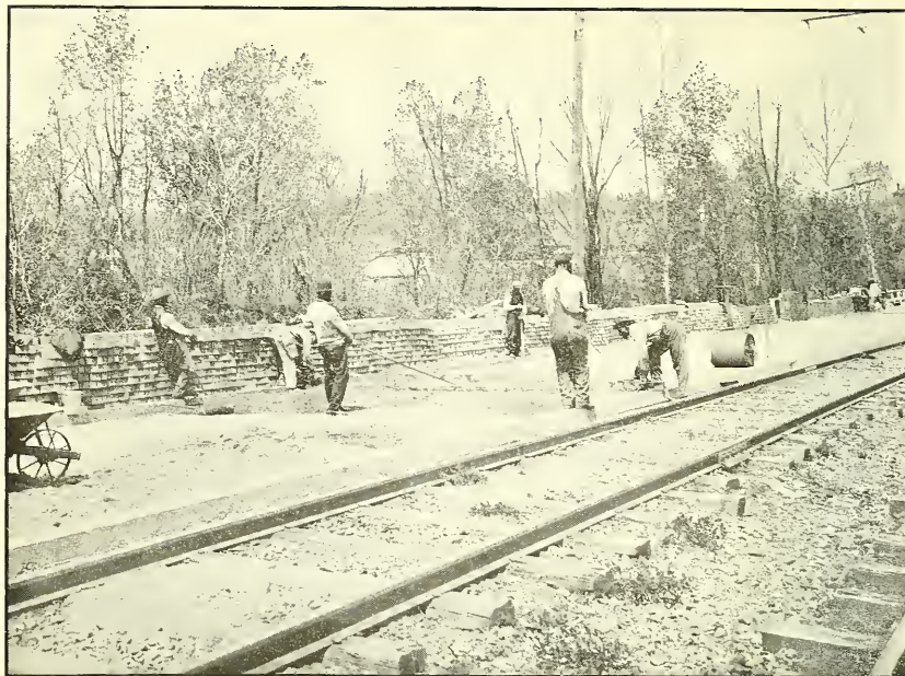
FIG. 1.—SPREADING SAND CUSHION.
