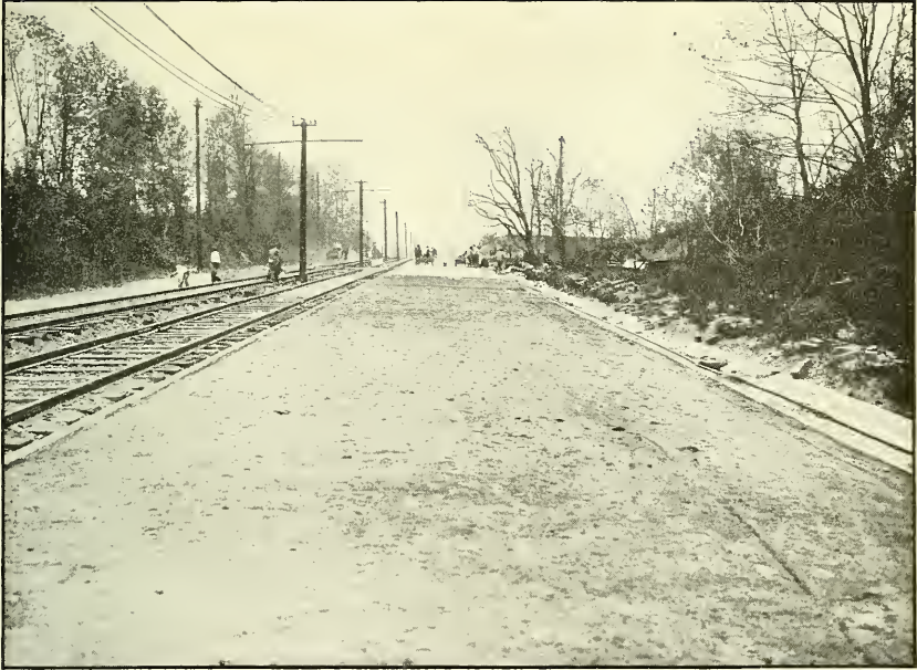
FIG. 1.—FINISHED BRICK PAVEMENT PROTECTED BY SAND COVERING.
