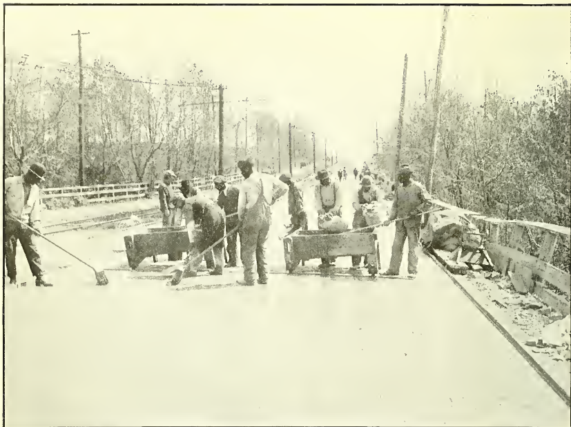
FIG. 1.—FILLING THE JOINTS, FIRST COAT.
