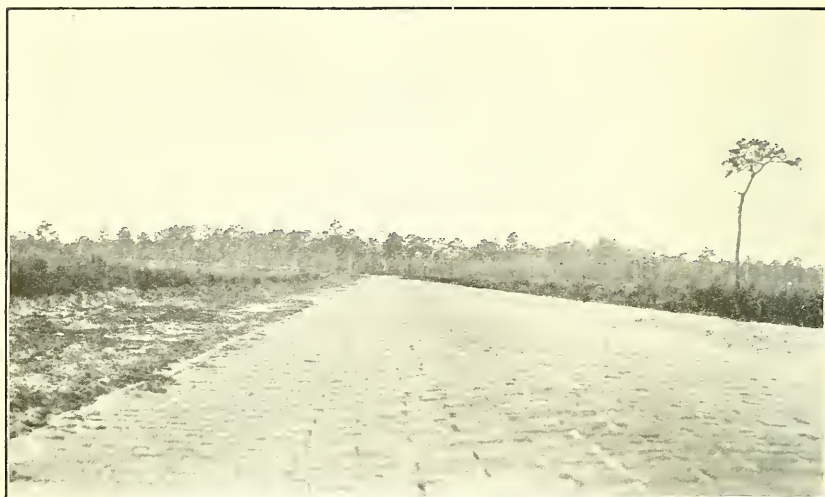
FIG. 1.—BRICK ROAD ON SAND FOUNDATION, HILLSBORO COUNTY, FLA.
