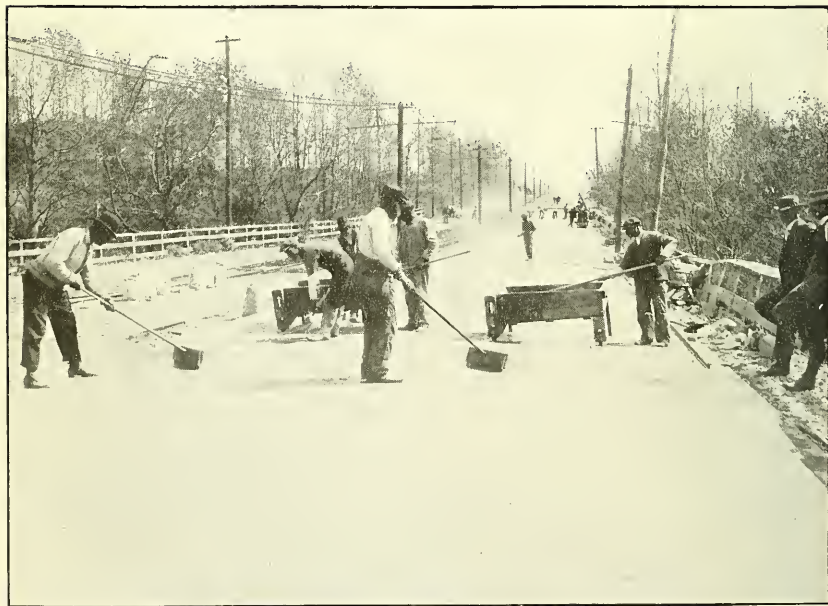
FIG. 2.—FILLING THE JOINTS, SECOND COAT.
