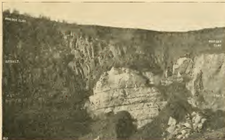
FIG. 1.—Columnar Basaltic Lava-flow, resting upon old land-surface of denuded Chalk. Quarry at Whitehead, Belfast Lough. Typical Section in the Antrim Plateaux. The lava has been subsequently denuded, and boulder-clay has been deposited across the whole. Photographed by Mr. R. Welch.
