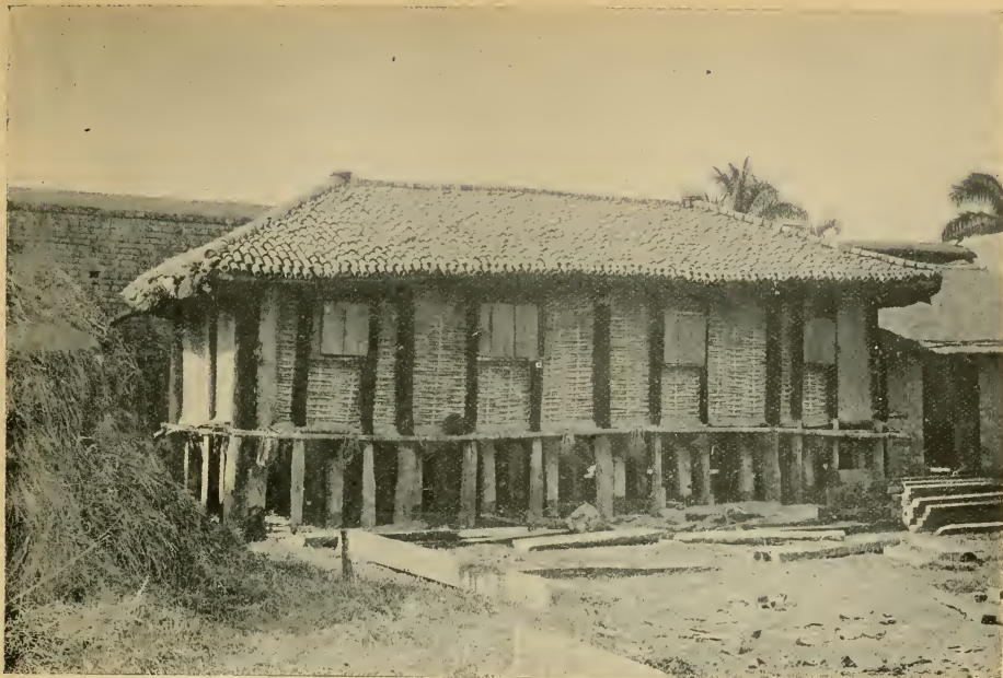
Fig. 1.—A Bakhari under construction and almost completed. The walls, of bamboo wattling, have not yet been plastered with mud.
