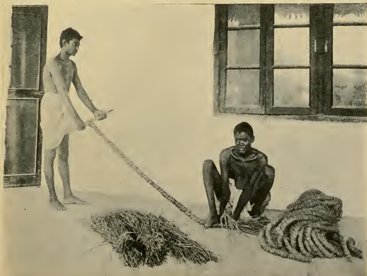
Fig. 2.—Preparing a straw rope for building a Morai . It is fed with the right hand and twisted with the right foot of the feeder, and twisted with the hands of the twister.
