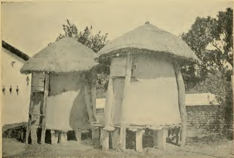
Fig. 2.—Two Bakharis of a type used in Bihar for storage of grain.
