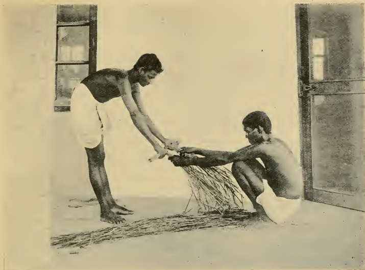
Fig. 1.—Commencing a straw rope for the building of a Morai .
