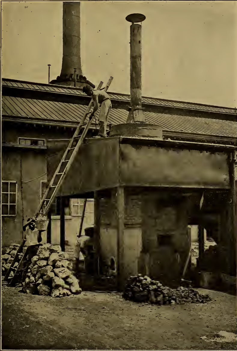
PLATE I. FIRST LIME KILN BUILT BY THE BUREAU OF SCIENCE.
