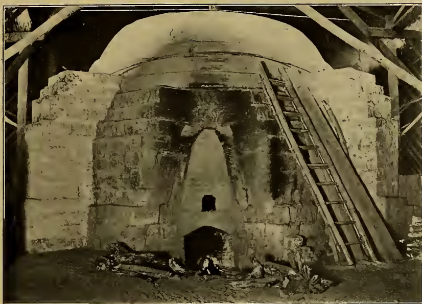
Fig. 1. Kiln at San Pedro Macati brick factory.
