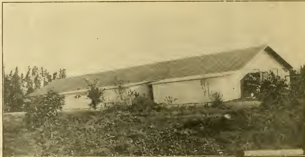
PACKING SHED, BUILT OF ADOBE, OF CHASE ROSE COMPANY, RIVERSIDE, CAL.
