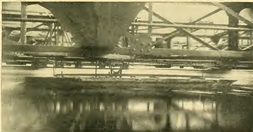
FIG. 2.—Model being towed—showing waves created.
