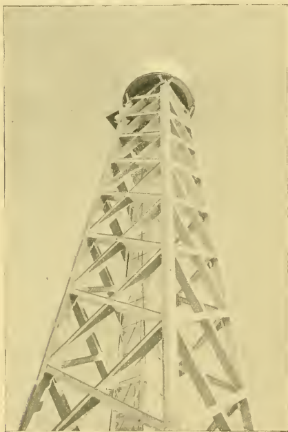
FIG. 1.—The tower telescope as seen from immediately below, showing the platform and dome at the top.
