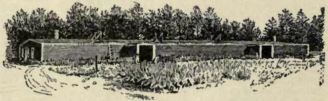
2404. A half-cellar storage.
