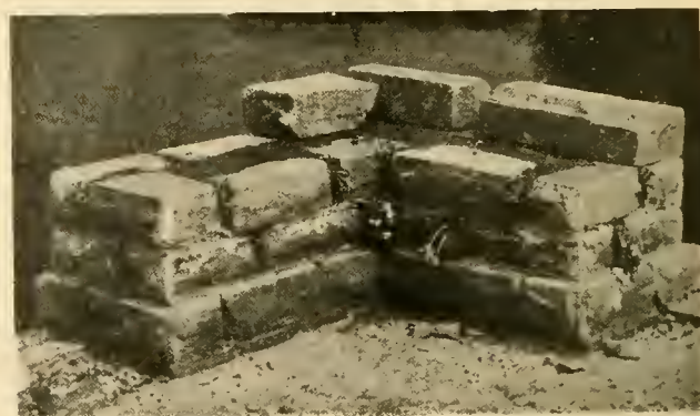
1.—A SMALL PILLAR IN THE COURSE OF CONSTRUCTION.
