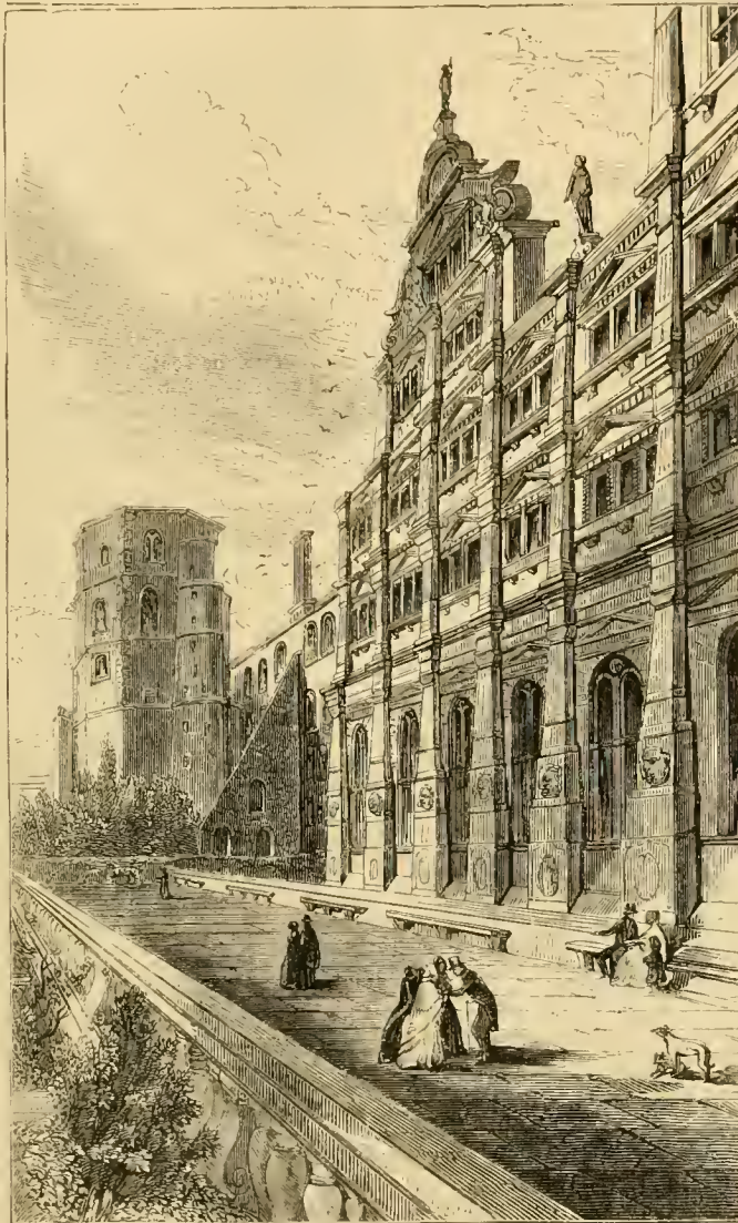
THE TERRACE AT HEIDELBERG.
