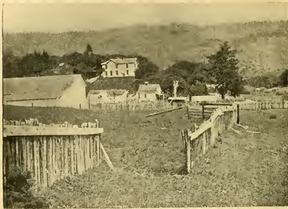
FIG. 1.—Fence parted by Earthquake Fault. The fault trace or fracture accompanying the earthquake is inconspicuous although the horizontal displacement is considerable. (Photograph by G. K. Gilbert.)
