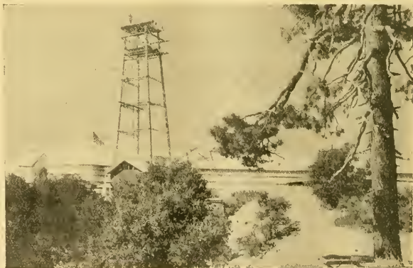
FIG. 2.—Vertical Cylindostat or Tower Telescope, Mount Wilson Solar Observatory.
