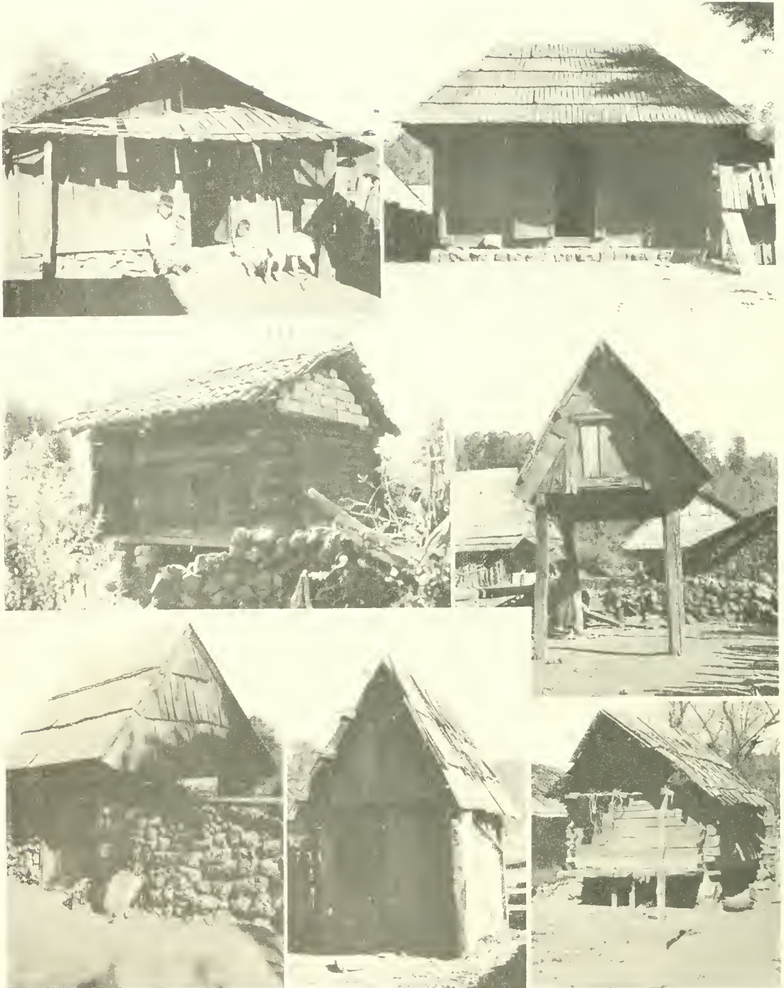
Upper (left) Kitchen of simple type with cogee posts (Angahuan). Upper (right) Kitchen of elaborate type (Angahuan). The gate and half door is here in Chocoma. Middle (left) Wooden "traje" at Ihuatzi, Lake Patzeuano, with tile roof and adobe support for the cogee posts. Middle (right) Storehouse of style found mainly in Angahuan (tmutakata). Lower (left) Large storehouse (tmutakata) over gate. Lower (center) Storehouse (tmutakata) with lower part made into a room. Lower (right) Storehouse (tmutakata) Chocoma.
