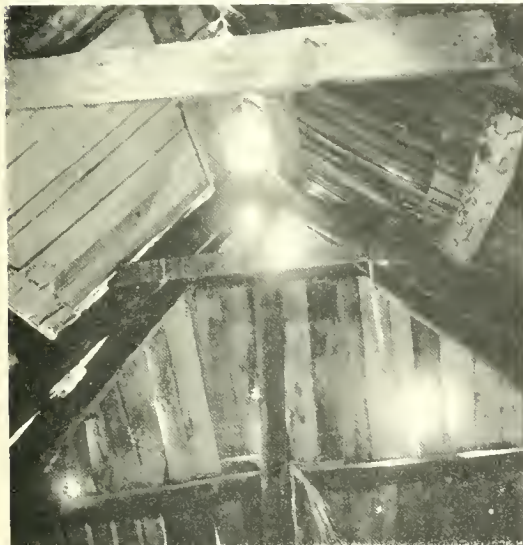
Upper (left): Simple kitchen under construction in Cheran, "pie derecho" type. Upper (right): Two roof sections in place in process of moving a Cherán house. Lower (left): Arrangement of rafters in Paracho house without ridge pole. Lower (right): Old house in Paracho of unusual style. The elaborate carving and absence of capitals of the pillars should be noticed. The walls are of vertical planks rather than the normal horizontal construction.
