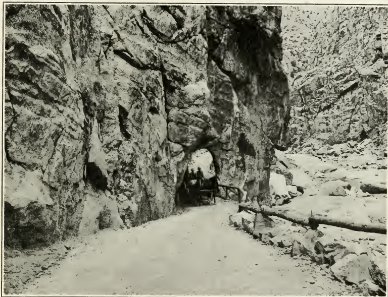
Detail View of Complete West Entrance of Tunnel just below Shoshone Dam Site on Canyon Road, Shoshone Project, Wyoming
