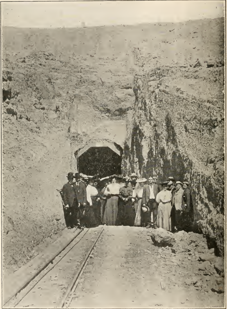
Congressional inspection party at the mouth of the Gunnison Tunnel, Colorado, now 7,000 feet within the mountain. One of the most interesting engineering projects the Reclamation Service is engaged upon.
