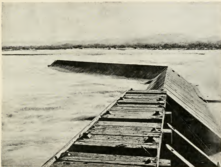
View Showing the Remaining Portion of the Arizona Dam, which was Washed Away by the Flood of April 13, 1905.
