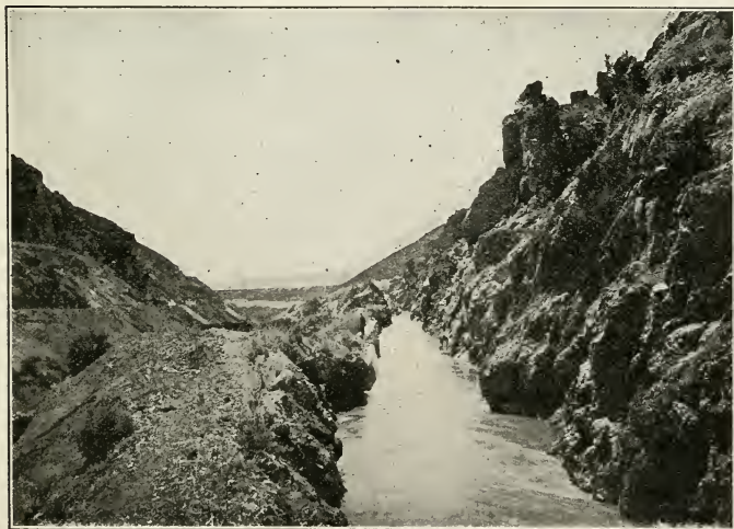
Section of Turlock Canal, California.
