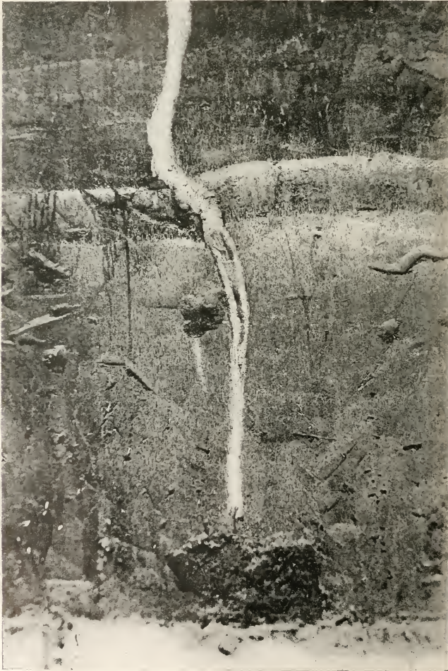
Fig. 1—Earthquake crack filled with sand forced up from below during New Madrid earthquake, Charleston, Mo. (Photo loaned by Mr. Thomas Beckwith.)
