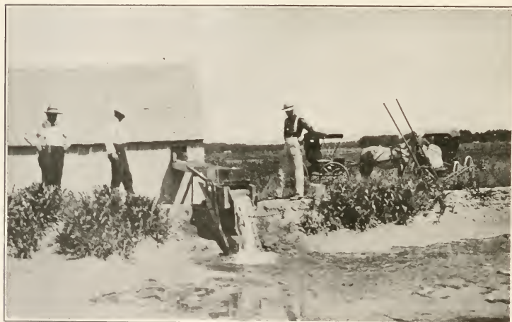
Fig. 4—Measuring weir at pumping plant near Garden City, Kansas. At the time the photograph was taken the pumping plant was yielding 200 gallons of water per minute
