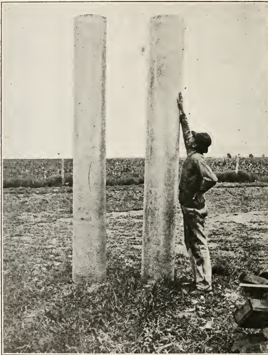
Fig. 1—Well strainers made of slotted galvanized iron. These strainers are 15 inches in diameter, and ten feet long, provided with 3-16 by 1 1-4 inch hit and miss slots, punched before the steel is galvanized. The strainers shown in the diagram were made of No. 18 wire gage sheet steel.
