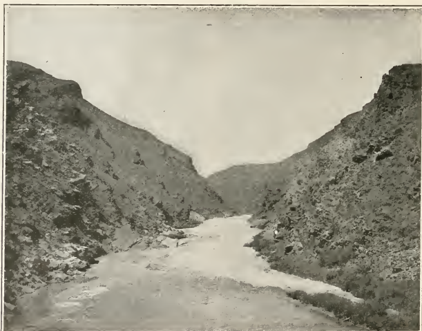
Salt River Canyon, Arizona, Looking Down Stream from Point About Half Mile Above Dam Site.
