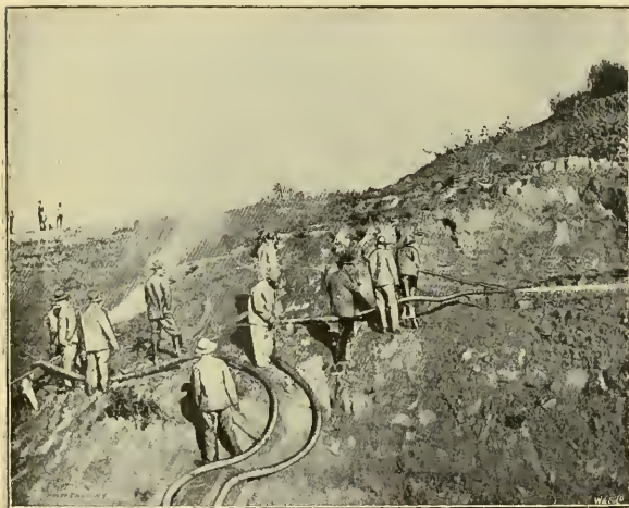
FIG. 1.—Details of Hydraulic Grading.
