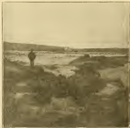
FIG. 2.—Broken roadway, with meadows submerged by the peat-flow, at Annagh Bridge. Foreground of heaped-up peat-mud and hog-timber. Lymne's cottage in the distance.
