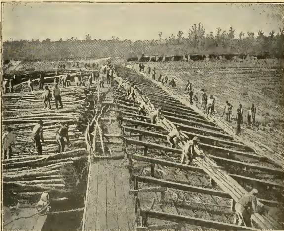
FIG. 2.—Constructing Fascine Mat on Mattress Ways.
