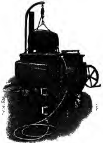
ROAD TAR SPRAYING MACHINE.
