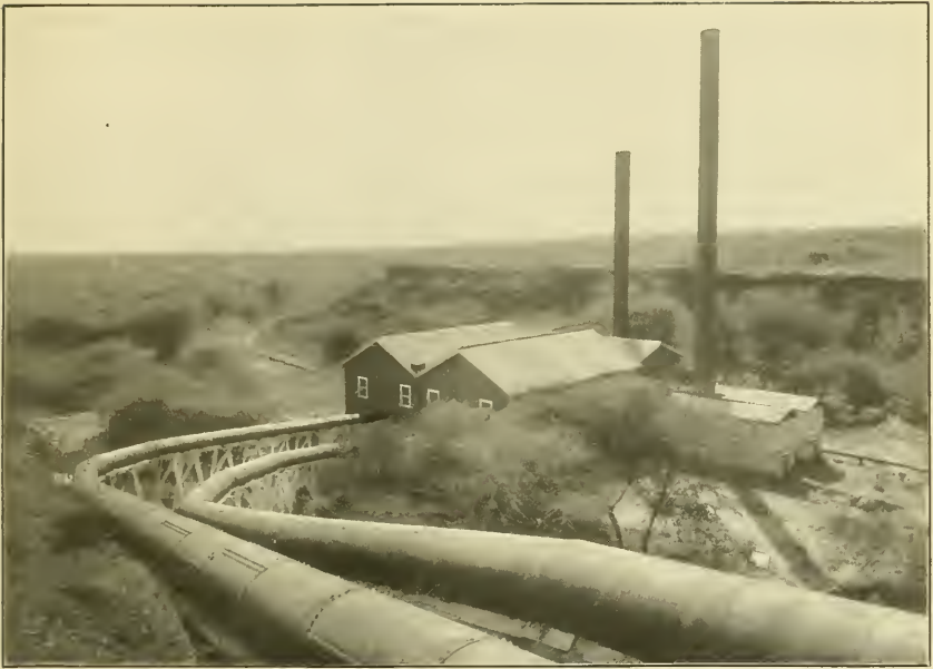
FIG. 1.—EWA PLANTATION PUMPING STATION.
