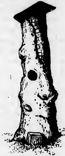
DECAYED ASH AND BRICK.
