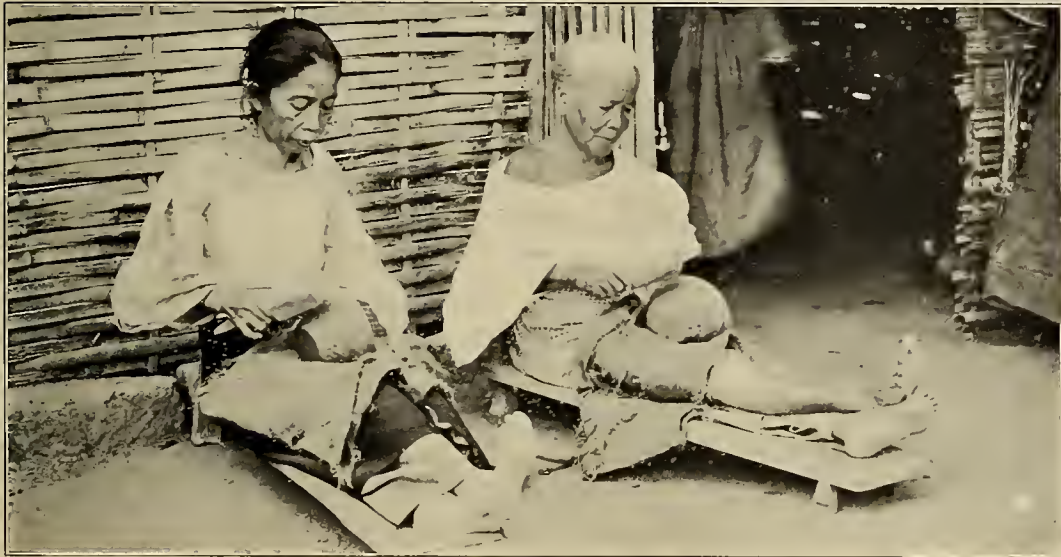
FIG. 2. BEATING POTS INTO FINAL SHAPE.
