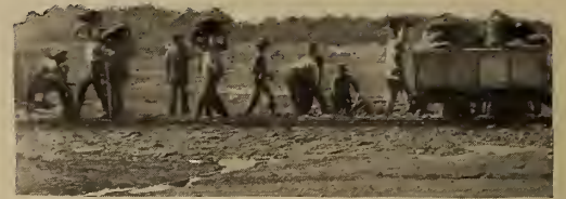
Natives digging and loading asphalt at Trinidad Lake
