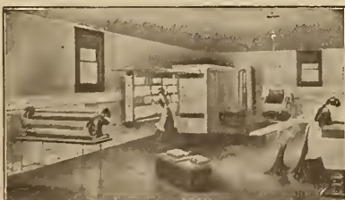
A Modern Residence Laundry Room showing installation of "CHICAGO-FRANCIS" Dryer and Laundry Stove
