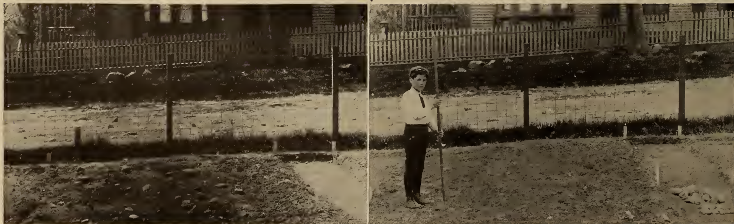
Begin work by clearing the garden of all rubbish and stones, placing them first of all in the path, to remove later
