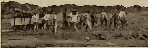
Busy asphalt-diggers in Trinidad Lake
