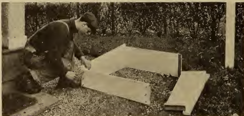
The Junior frames are next in size to the melon and take a sash 34 x 38 inches. We make them for one, two, three or any number of sash.
