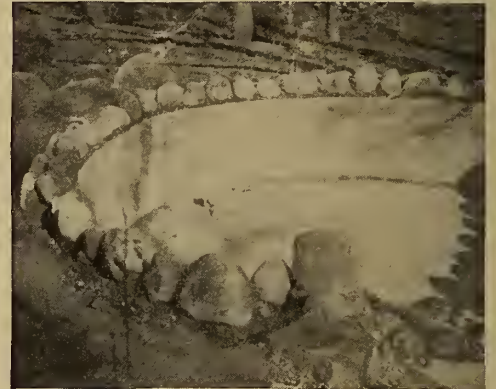
The finished pond, fed by an artificial brooklet and drained by underground tile
