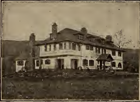
Residence of Thomas Shields Clarke, Esq., Lenox, Mass. Stained with Cabot's Shingle Stains and lined with Cabot's Sheathing Quilt for warmth. (See letter.) Wilson Eyre, architect, Philadelphia
