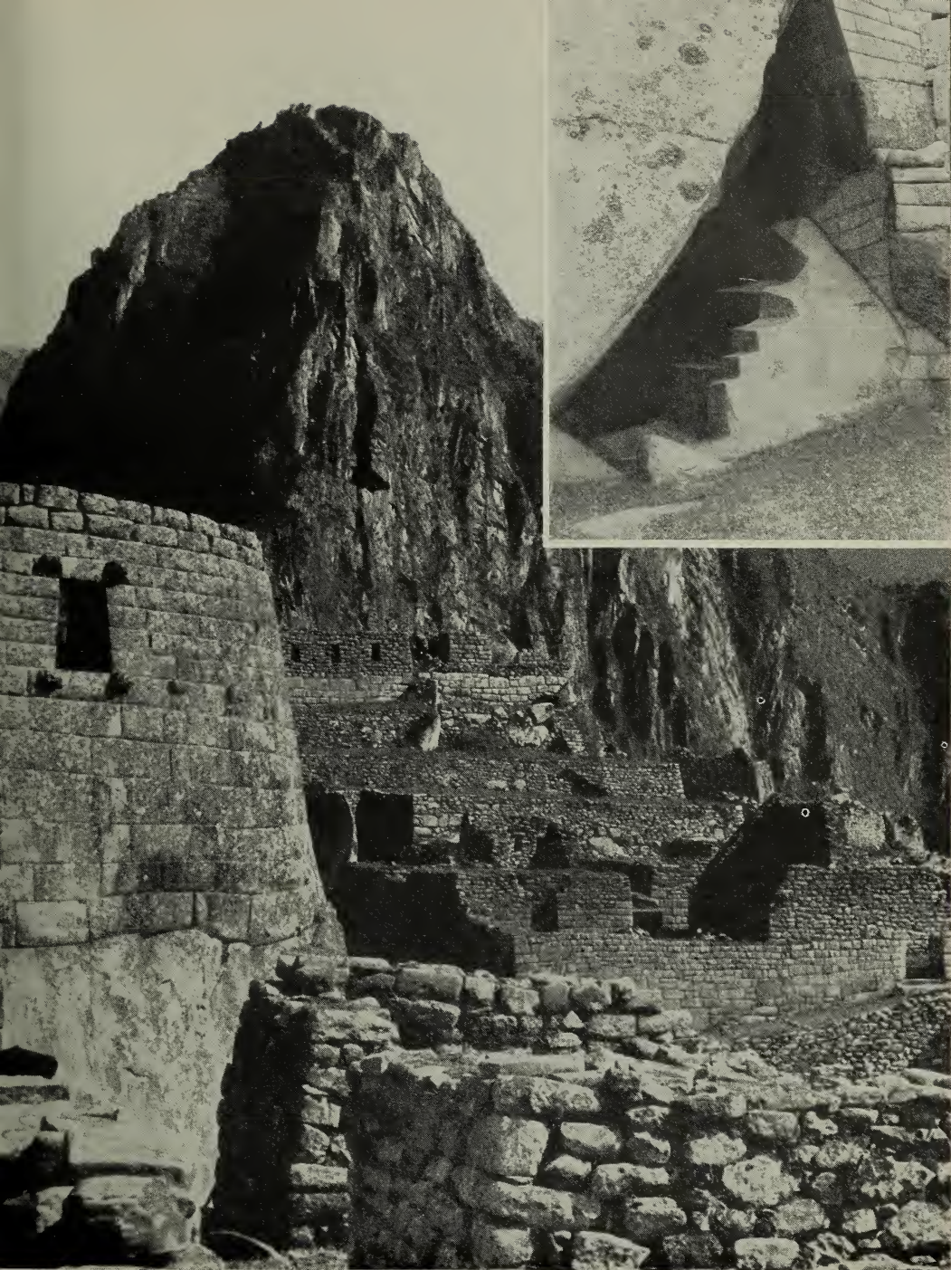
PLATE 81.—Machu Picchu stone masonry and architecture. Top (right): Monolithic carving combined with ashlar masonry. (Courtesy Truman Bailey.)
