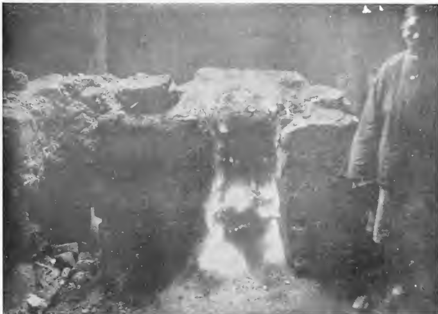
FIG. 1. LOW IRON FURNACE OF THE TIEN-TAUNG KUAN IN BLAST.
