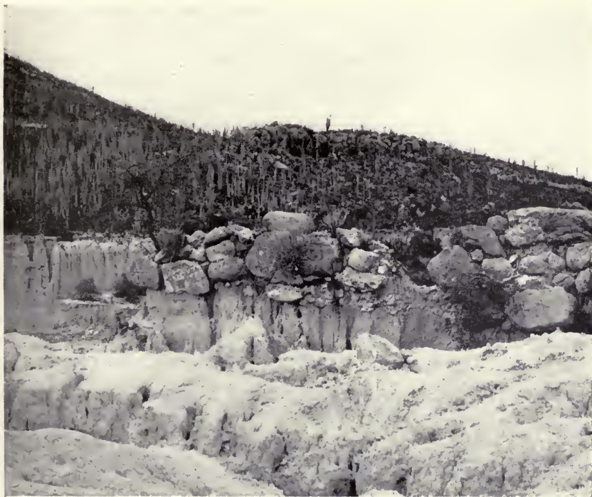
FIG. 20. The remains of an ancient check dam near Teloxtoc in use during the Classic (Palo Blanco) period. Erosion has since deeply gullied the foreground and dug an arroyo 12 feet deep along the main watercourse.
