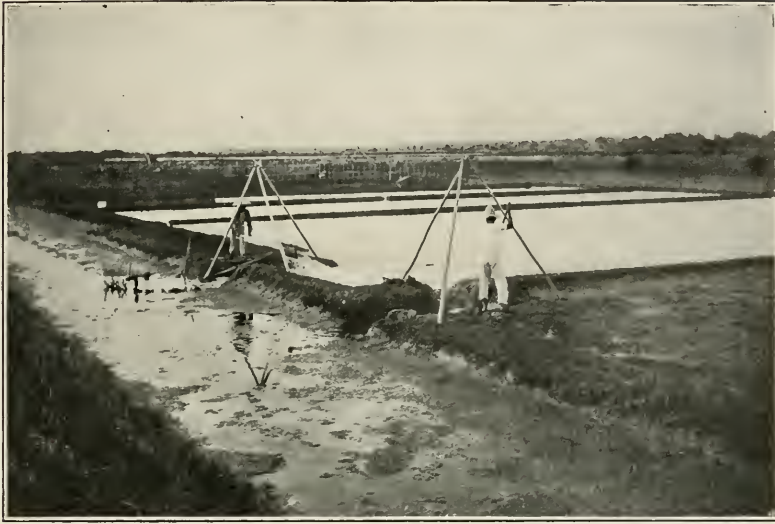
Fig. 1. Showing the apparatus for transferring brine from evaporating reservoirs to crystallizing vats which are on a higher level.
