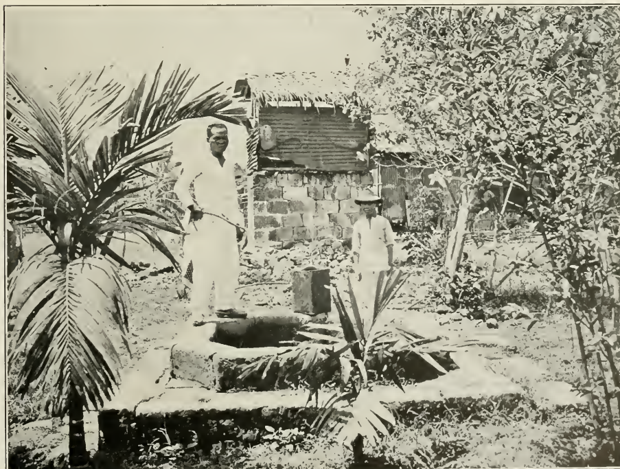
Fig. 2. Outhouse in proximity to well.
