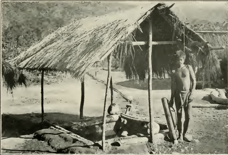
Fig. 2. The lower end of a bamboo trough from the Salinas salt springs, showing the well from which the brine is carried to the evaporating pans.
