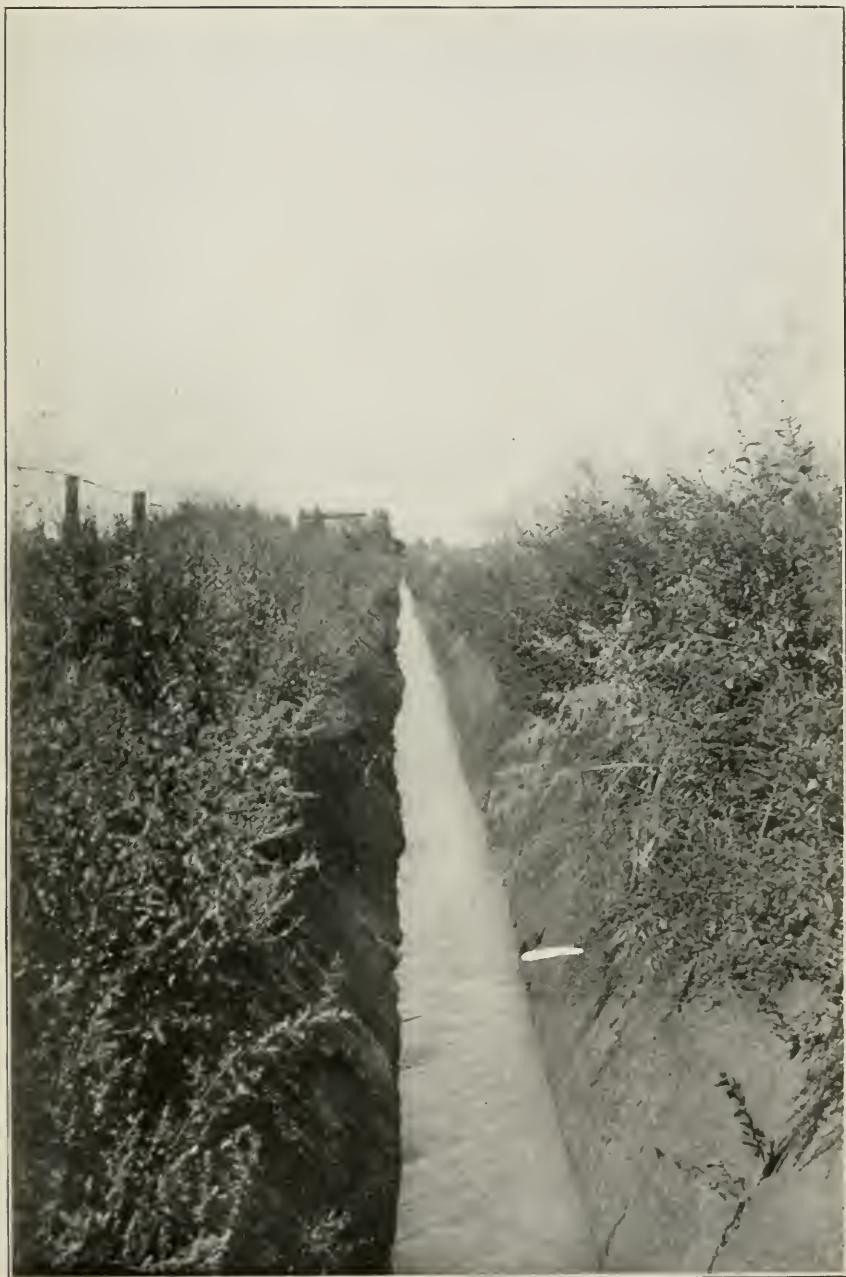
IRRIGATION INVESTIGATIONS—DRAIN DITCH FOR REMOVAL OF SEEPAGE WATER AND ALKALI FROM A HOP YARD.
