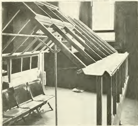
Exhibit of Cypress Construction by the John C. Moninger Co., and the Garland Iron Gutter by Geo. M. Garland, at the Buffalo Convention.
