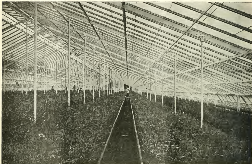
Iron Frame Carnation House, 306x51 feet, erected by Hitchings and Co. at Briar Cliff Farms, Sing Sing, N. Y.
