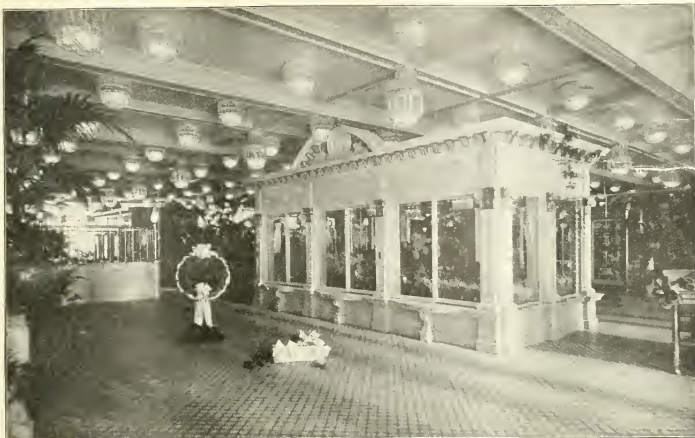
View in Fleischan's New Store, Chicago.
