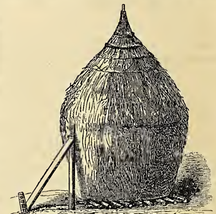
A STACK BRACED TO PREVENT LEANING.
