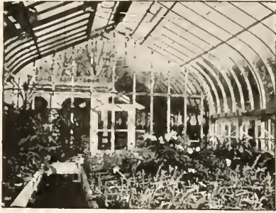
This interior view gives an idea of the lightness, airiness and construction of the Semi-Curvilinear type of
