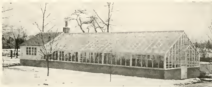
The greenhouse portion is 18 feet wide and 33 feet long.
