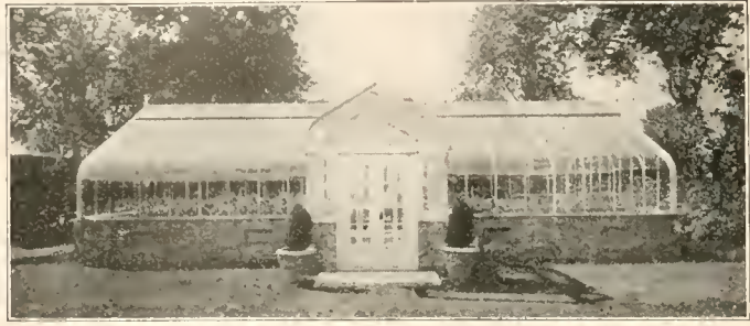
V-Bar Greenhouse Built for Louis B. Tim, Long Branch, N. J.
