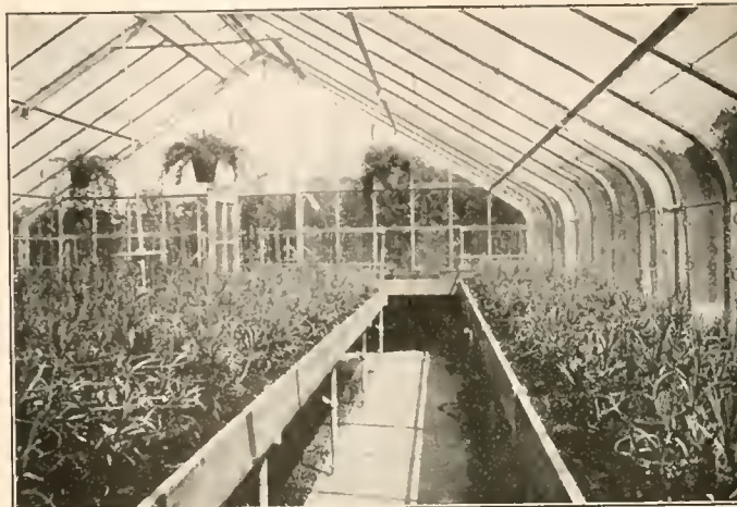
Interior of Patented V-Bar Greenhouse Erected on the Estate of Mr. Carl Tucker, Mt. Kisco, N. Y.
