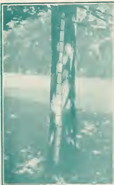
An example of sectional filling work done by Davey Tree Surgeons on the Mrs. L. M. Sargent estate
