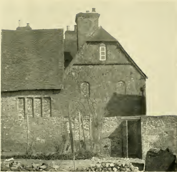
West side showing the blocked windows
