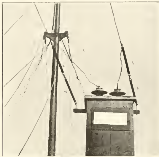
FIG. 2. SHOWING HARD RUBBER INSULATORS.
