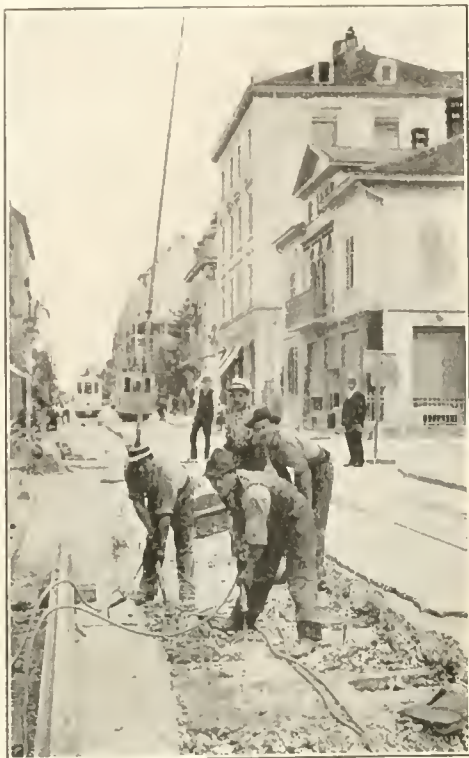
PNEUMATIC HAMMERS CUTTING CONCRETE.
