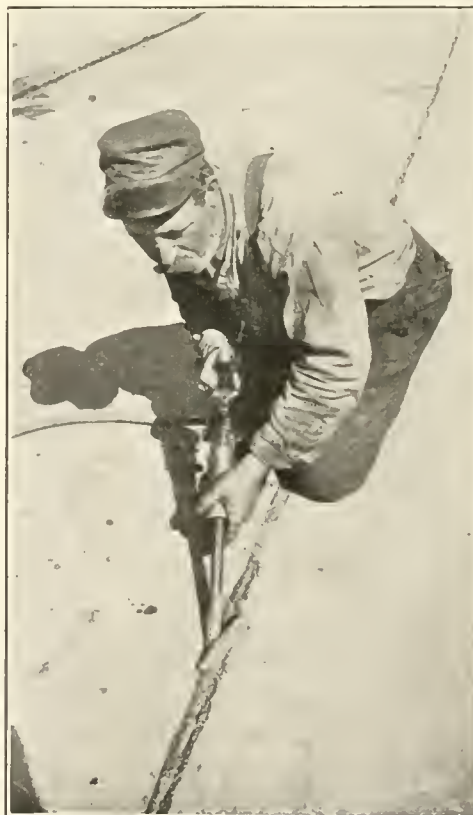
CUTTING ASPHALT BY COMPRESSED AIR.
