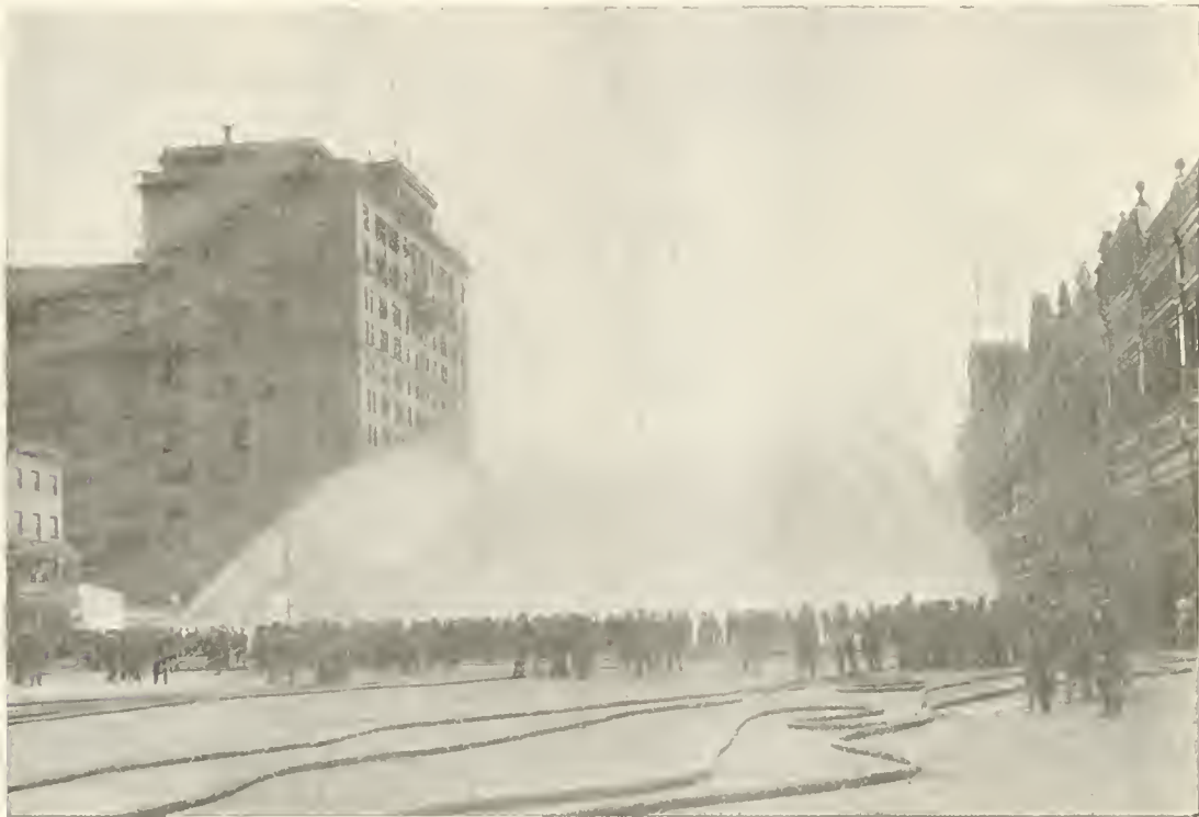
CAPACITY TEST, HIGH PRESSURE SYSTEM, NEW YORK.
