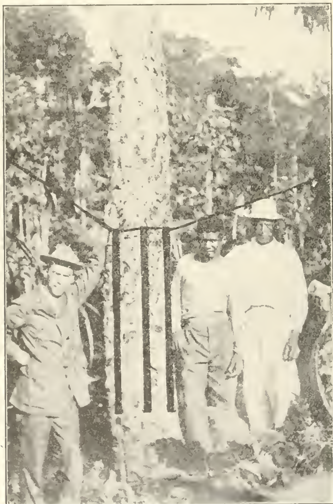
ELECTRICAL TAPPING DEVICE ATTACHED TO A RUBBER TREE.
