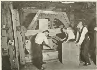
TESTING LAMP CONTAINERS IN SIX-FOOT DRUM.
