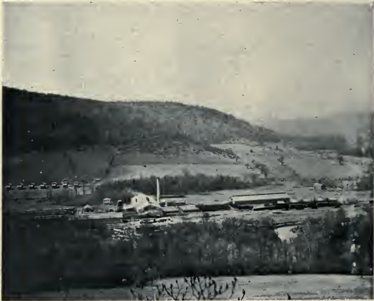
FIG. 56.—General view of hardwood distillation plant at Betula, Pennsylvania. On the left is the wood yard, in the center the oven house and still house and on the right, the charcoal storage warehouse. Immediately to the right of the oven house are the two sets of cooling ovens.
