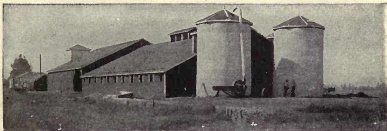
FIG. 29.—A California dairy barn, with concrete silos, each 15 ft. diameter by 30 ft. high; capacity, 100 tons.
