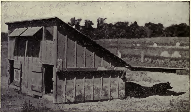
FIG. 83.—Portable hog-houses with low, flat roofs; if used for housing swine in hot weather, they should be provided with a shade at the rear under which the pigs can lie in comfort. This shade is five feet wide, made of inch stuff placed upon removable supports which rest upon cleats nailed to the ends of the house. (Wisconsin Station.)
