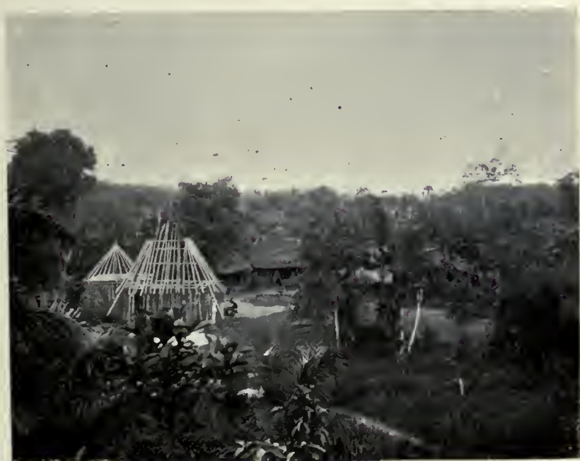
387. VAI HOUSES IN PROCESS OF CONSTRUCTION
