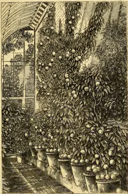
FIG. 288.—ORCHARD-HOUSE AT SCONE PALACE.
